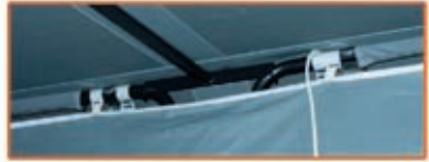
Savanne/Concorde: Mount the roof sup. pole.
